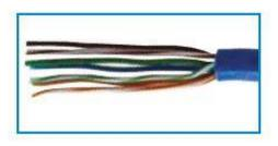
Step 3: Untwist pairs to jacket base, and align in order. Trim ends flat.
